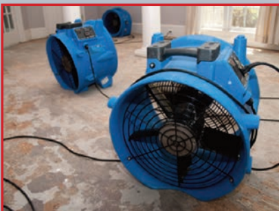
Check humidity and ambient temperature during restoration drying
