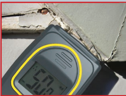
Check drywall for moisture
