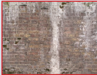
Check for moisture in masonry
