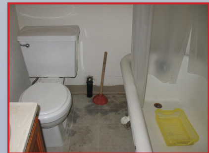
Locate moisture under bathroom floors
