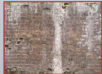
Check for moisture behind masonry
