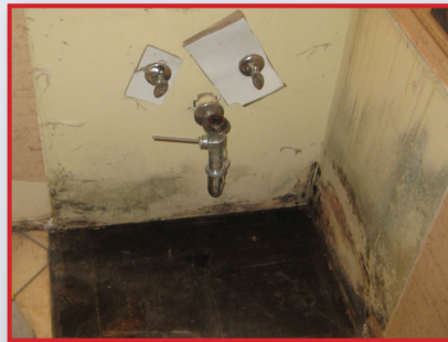
Locates moisture under bathroom vanities where mold thrives
