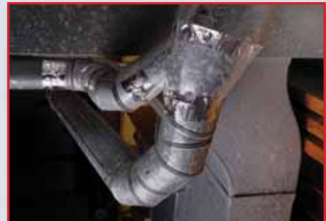
Minimally Invasive Duct Leak Testing
