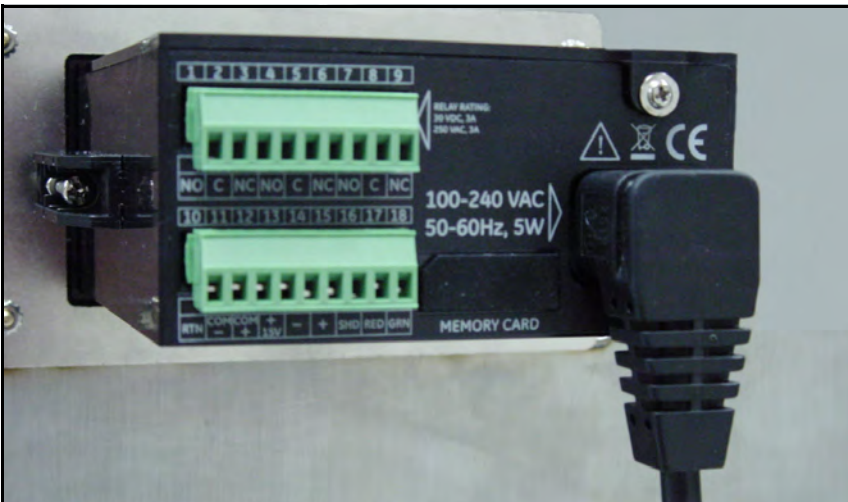
Figure 39: The AC Power Cable Installed
