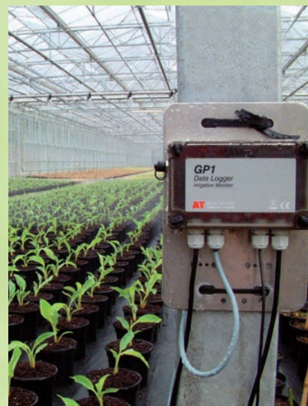
GP1 Data Logger controlling precision gantry irrigation within a glasshouse at Hillier Nurseries.
